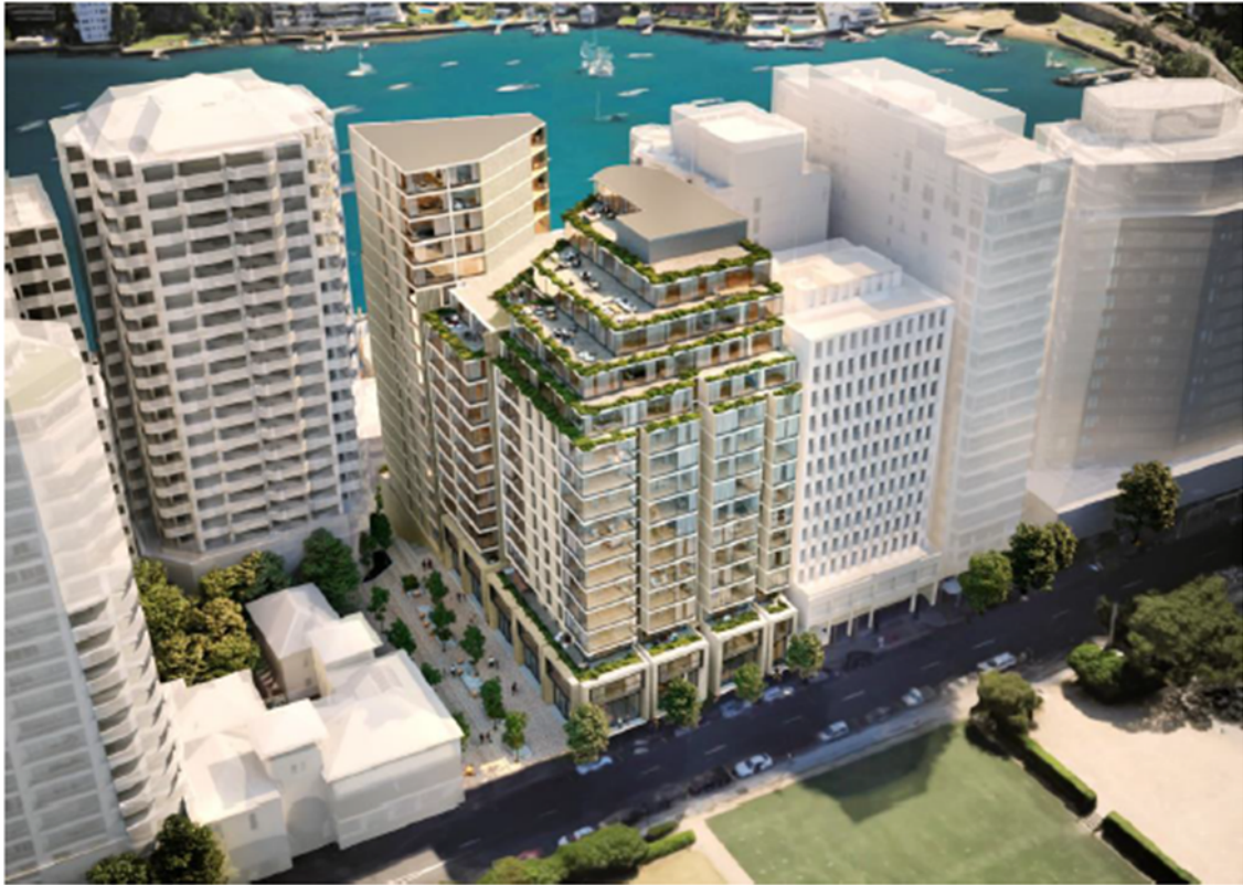
FIGURE 1: Reference design accompanying Planning Proposal for 52 Alfred Street South, Milsons Point (PP5/20).
