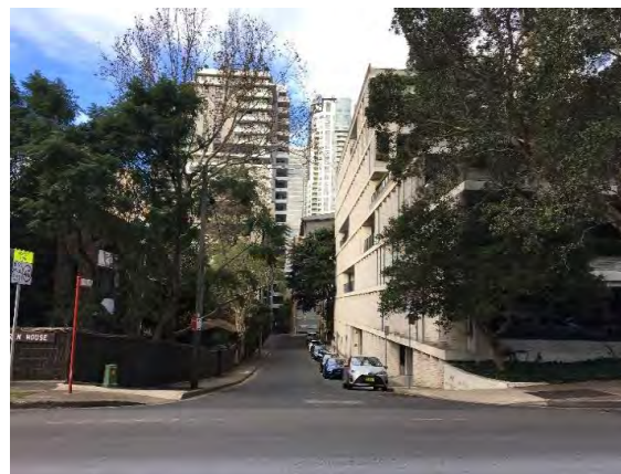
Picture 4: Site as viewed from the north-west, illustrating the relationship to Harnett Street
