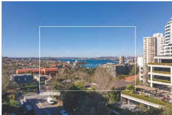
Picture 20: Existing view from RL92.36 (approximately L7) of the western stack of Aqualand
