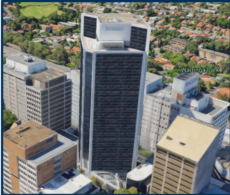
Figure 10 View of Tower to the south of the site at 141 Walker Street
