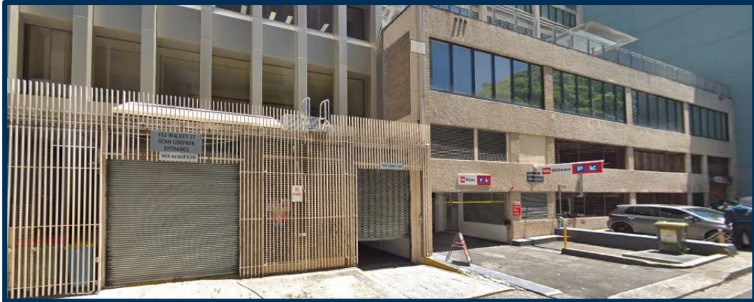
Figure 7 View of Little Walker Street Site frontage
