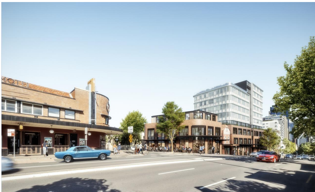
View looking south along Pacific Highway
