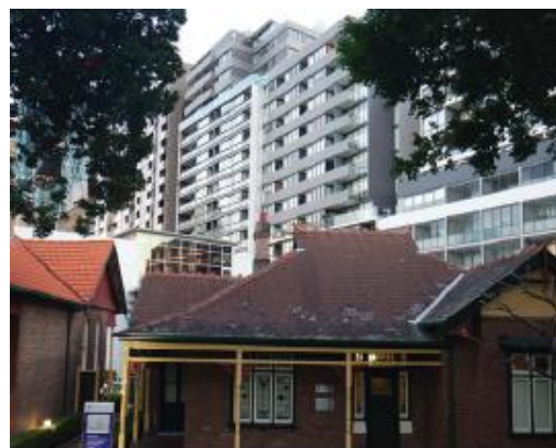
Recent development showing an abrupt edge to towers relative to low scale developments.
