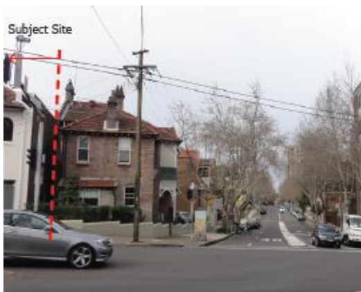
Existing 2-storey dwelling within the conservation area to the south.
