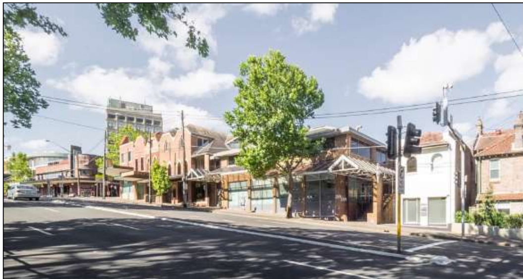
Photo 1: Existing commercial buildings fronting Pacific Highway
