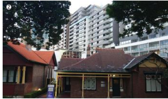
Recent tower development viewed from McLaren Street Conservation Area.
