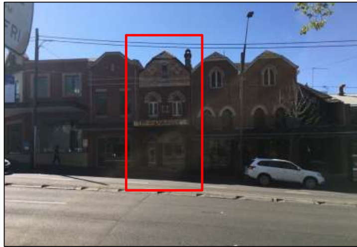
Photo 2: Existing Heritage building
