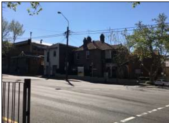
Photo 5: Contributory building at No 6-8 McLaren St
