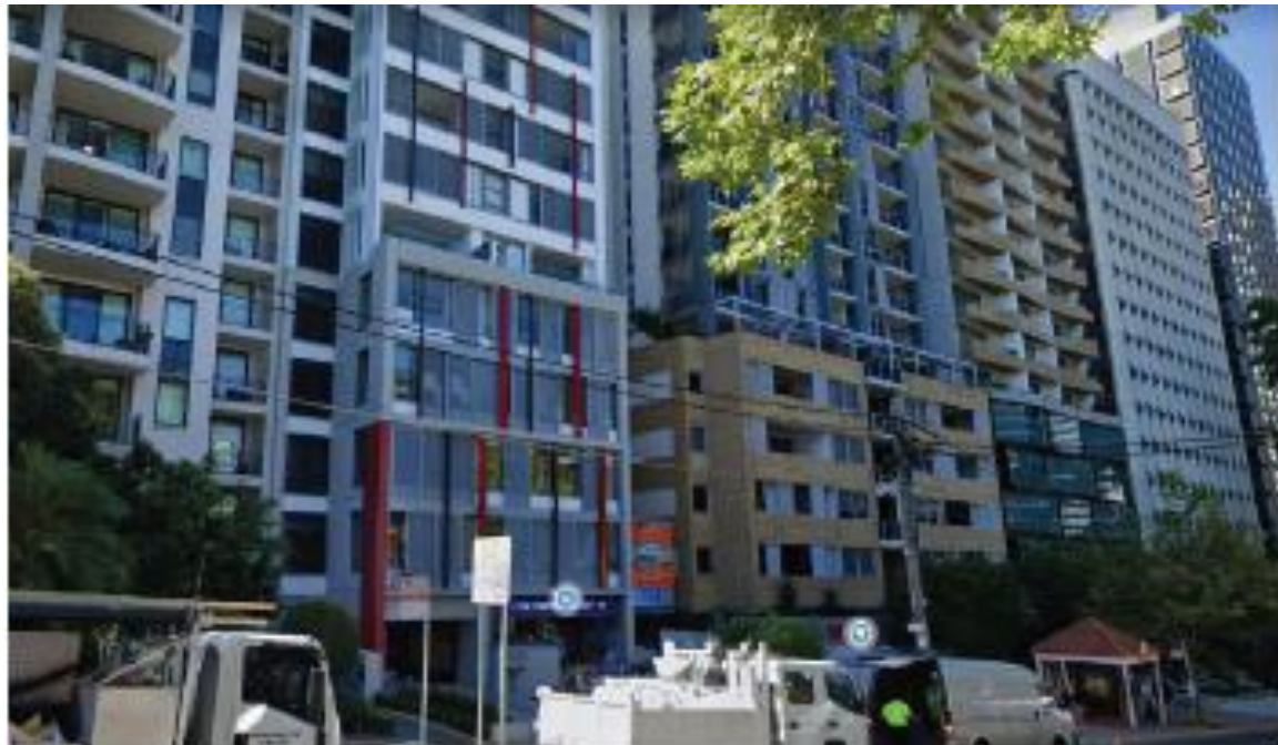
Figure 29 Recent Mixed-Use Tower Development along Miller Street
