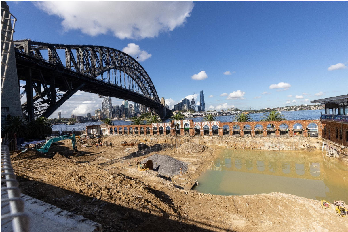
Lift Pit excavation 14/3/2022
