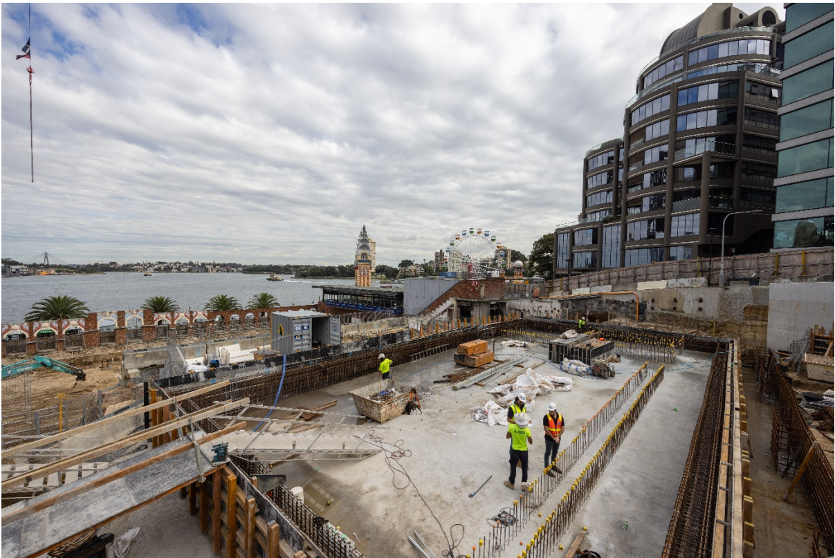
Program pool under construction 06/05/2022
