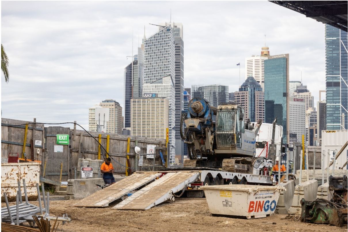
The piling rig arrives 06/05/2022
