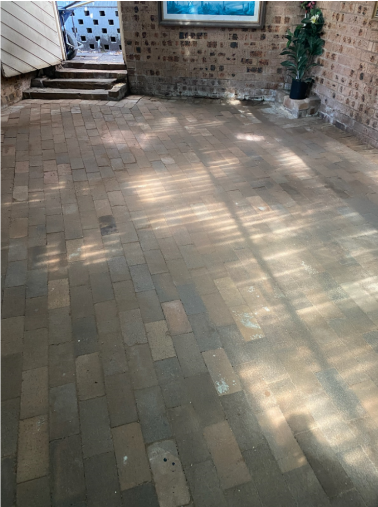
57 Ridge Street – North Sydney - courtyard pavers
