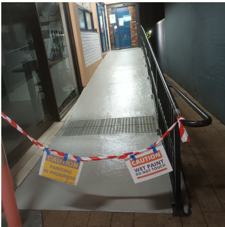
Neutral Bay Community Centre pedestrian ramp
