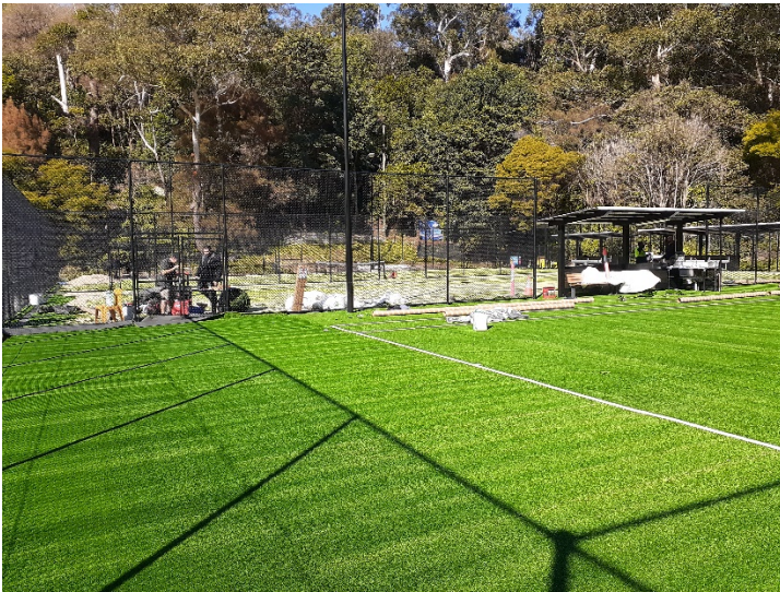
Primrose Park Tennis - Synthetic grass being laid
