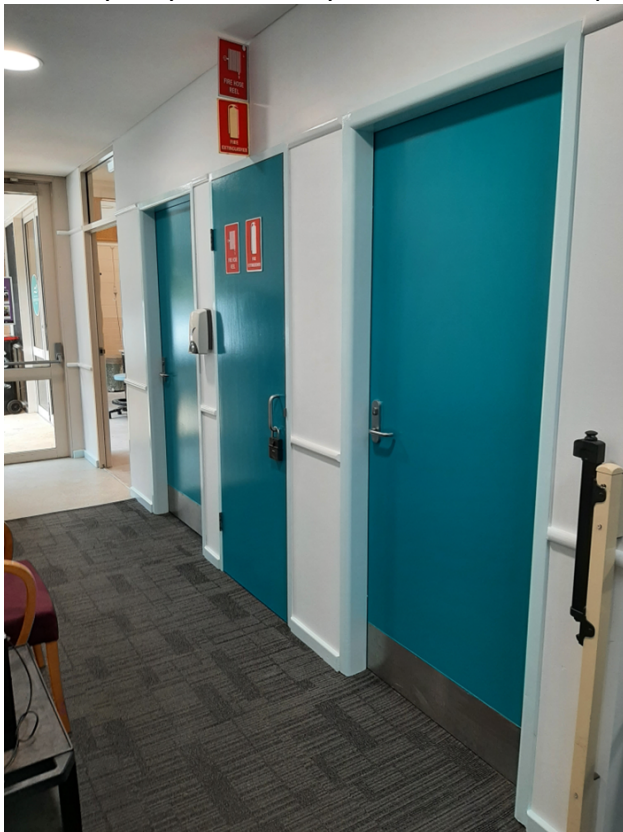
North Sydney Community Centre - internal repainting
