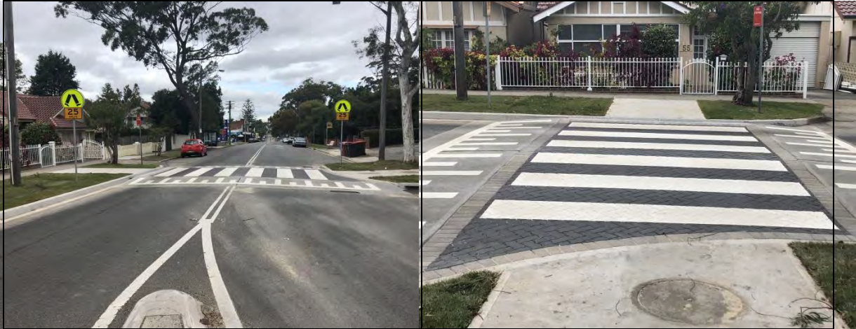
Pedestrian Crossing Upgrade – Spofforth Street, Cremorne
