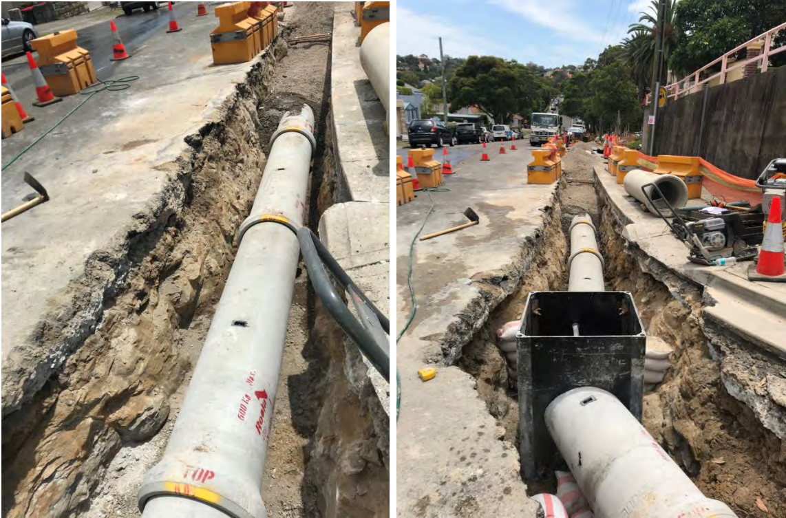
Pit and Pipe replacement at Milson Road, Cremorne Point.
