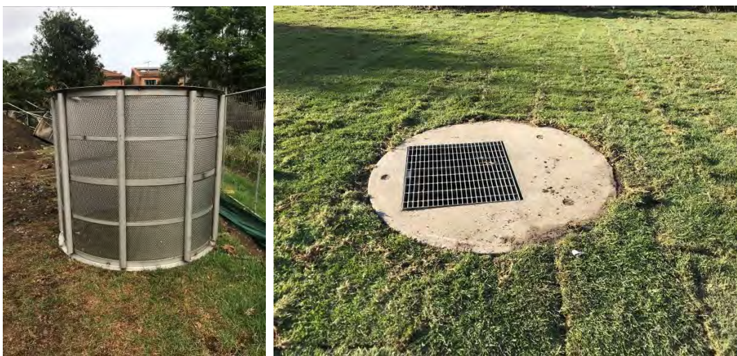
Replacement of GPT at Little Young St, Cremorne.
