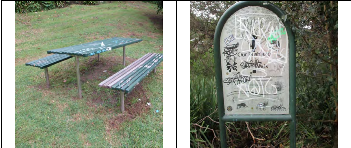
Examples of failed and failing Park Furniture, Playgrounds, Sporting Infrastructure assets in the North Sydney LGA
