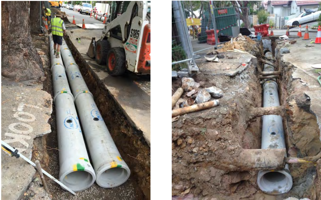
Pit and Pipe replacement at Carabella Street, Kirribilli.
