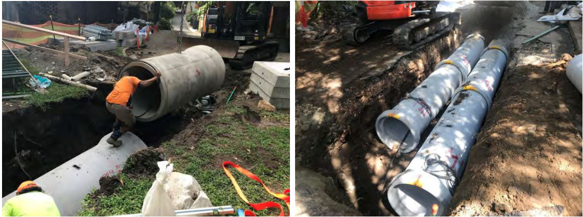
Pit and Pipe replacement at Carlyle Lane, Wollstonecraft.
