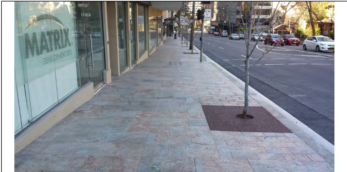
Pacific Highway, North Sydney – Granite
