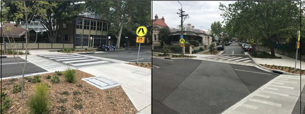
Pedestrian crossing improvements – McLaren Street and Church Street, North Sydney
