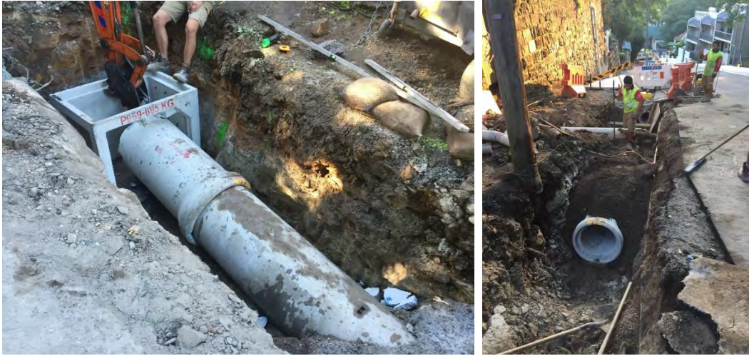
Pit and Pipe replacement at Bob Gordon Reserve, Lavender Bay.
