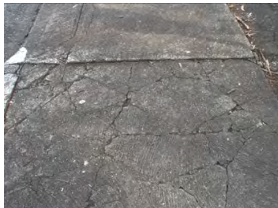
Concrete footpath in poor condition
