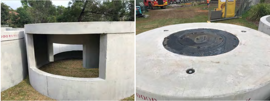
Replacement of GPT at Little Young St, Cremorne.
