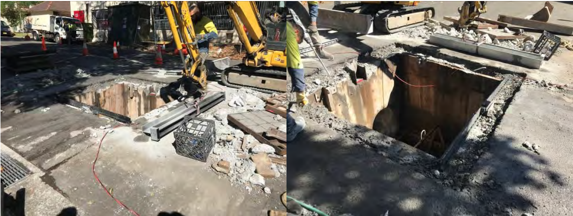
Replacement of GPT Lids at Elamang Avenue, Neutral Bay.
