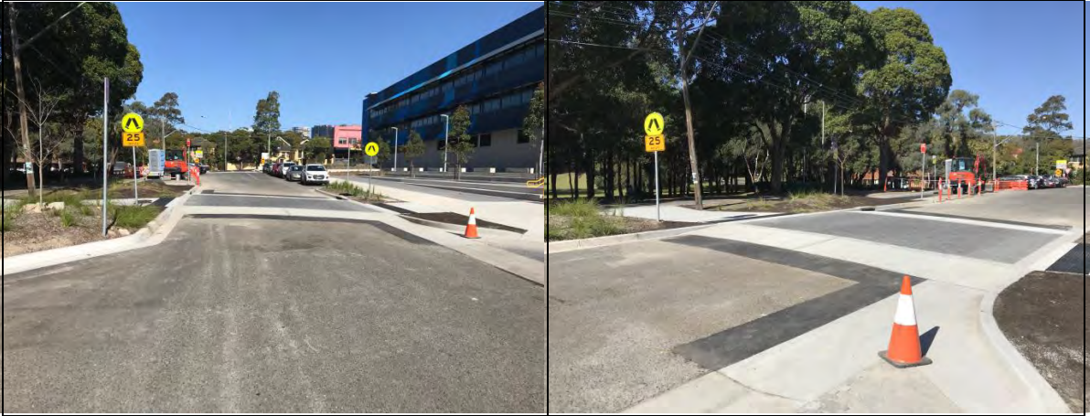
Pedestrian Crossing – Anzac Avenue, Cammeray
