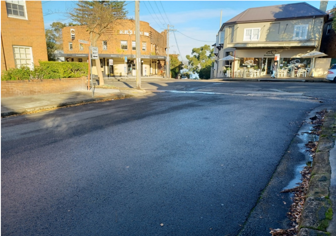
Photo 4. The existing site – 21/06/22
