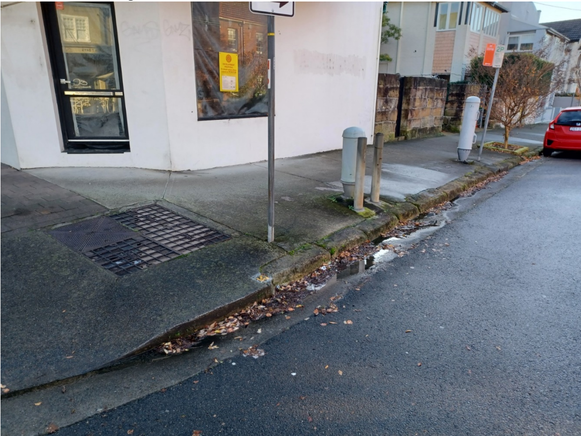
Photo 5. The existing site – 21/06/22
